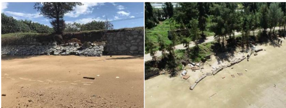
Figure 4. Seawall collapse and damage under storm surge and wave attack (Qinzhou Municipal Oceanic Bureau, 2021)
