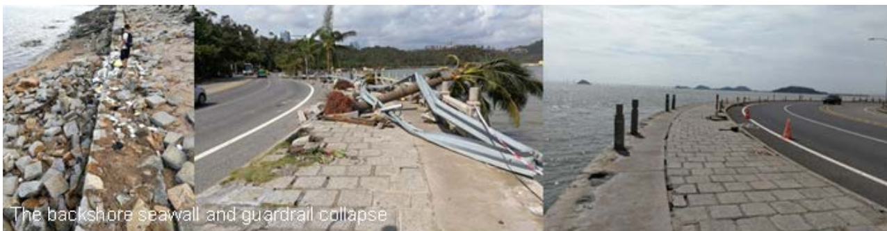
Figure 20. Coastal section without beach protection showing a collapsed seawall and damaged (Source: Third Institute of Oceanography, Ministry of Natural Resources)
