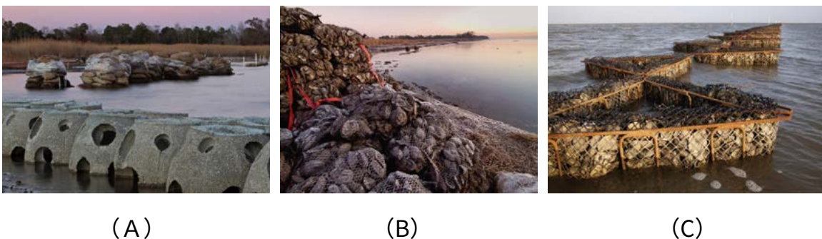
Fig.32: Oyster Reef Breakwater Construction in Alabama using (A) Reef Balls™, (B) Oyster Shell Bags, and (C) Oyster Cage Arrays (ReefblkSM), photo credit: (A) and (B) Erika Nortemann/TNC; (C) Beth Maynor Young.
