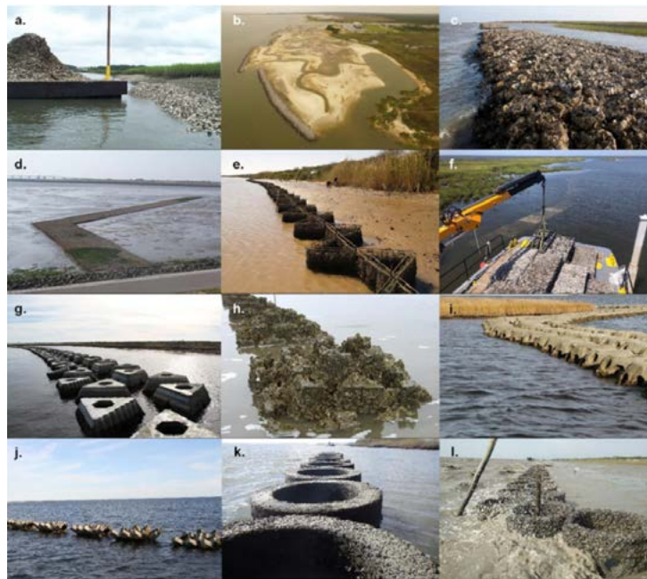
Fig.19 Oyster reef constructed in the intertidal zone for shoreline protection [12]
