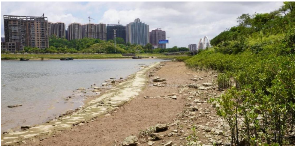
Figure 4 Schematic Diagram of Submerged Dam, with water channel at the outer side of the submerged dam and mudflat at the inner side of the submerged dam. (Wang Xin, 2021)
