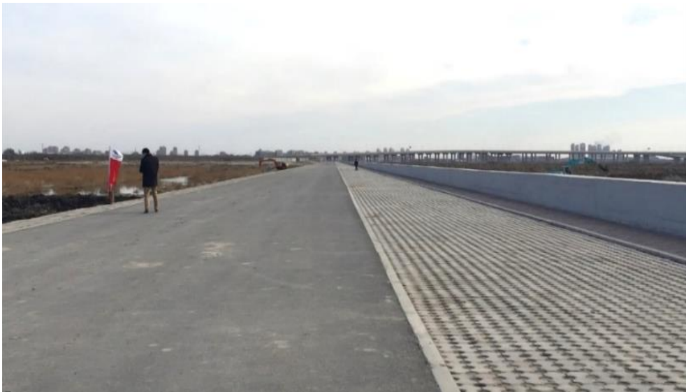
Figure 7: High Hard Protective Seawall Blocking the Land-Sea Connection. (China-Singapore Tianjin Eco-city Administrative Committee, 2016)
