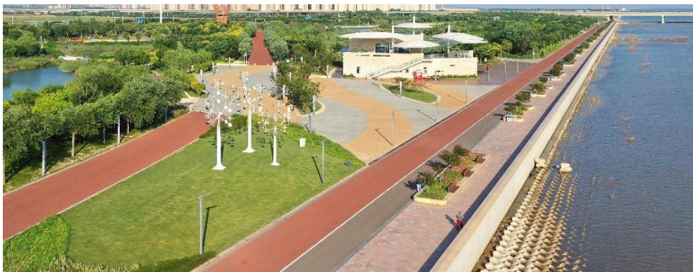
Figure 10 Coastal Greenway Mainly Reconstructed along Existing Seawalls. (China-Singapore Tianjin Eco-city Administrative Committee, 2021)
