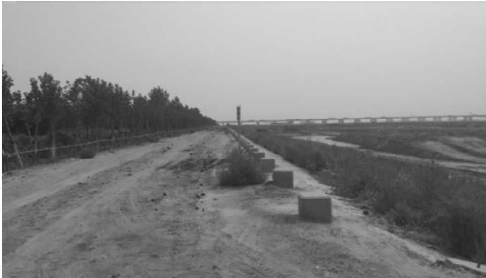
Figure 20 Before the Completion of Ecological Seawall Construction. (China-Singapore Tianjin Eco-city Administrative Committee, 2016)
