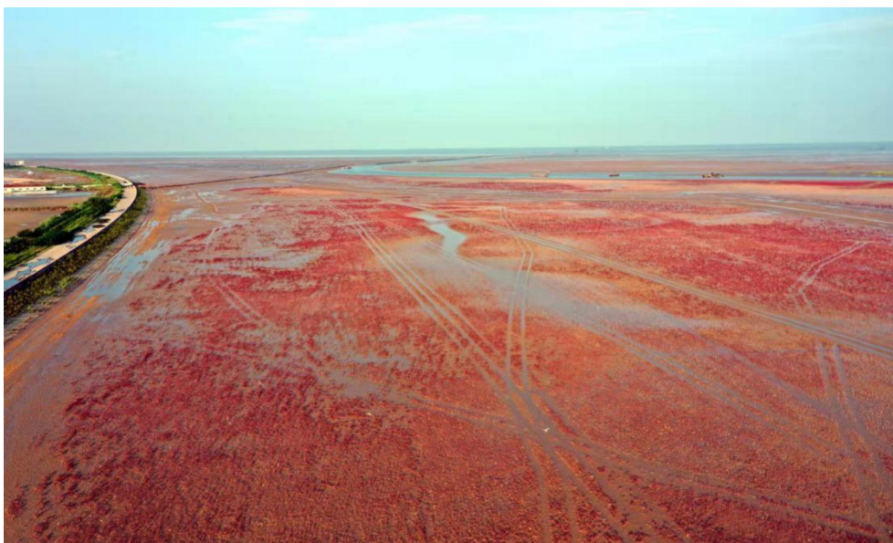
Figure 4 An integrated protection system of seawalls-vegetation-tidal flats. (Zhao Yingli, 2021)
