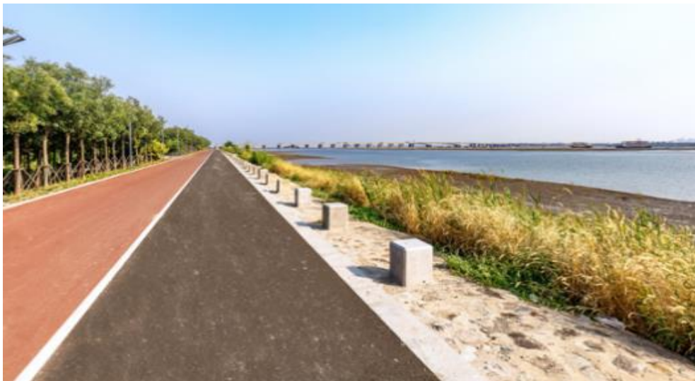
Figure 21 After the Completion of Ecological Seawall Construction. (China-Singapore Tianjin Eco-city Administrative Committee, 2021)
