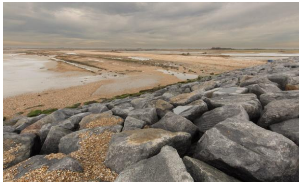
Figure 2 Rock revetment at seaward end of new embankment. (Harvey, 2021)
