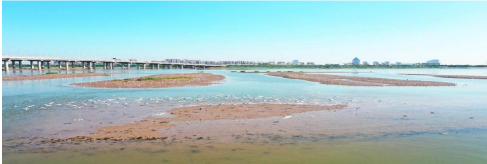
Figure 26 The Improved Wetland Environment outside the Seawalls after Construction. (China-Singapore Tianjin Eco-city Administrative Committee, 2021)
