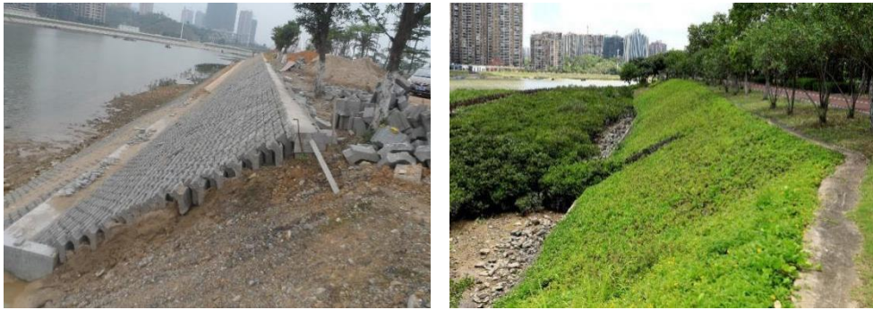
Figure 5 Before and After Construction of ArmorFlex on the Seawall. Left: Construction process of ArmorFlex (Wang Xin, 2015). Right: Seawall surface after planting vegetation (Wang Xin, 2021).
